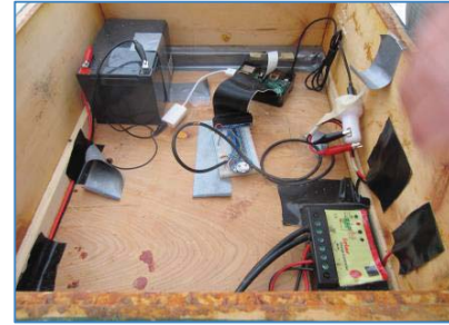
Figure 1. BeePi hardware components
