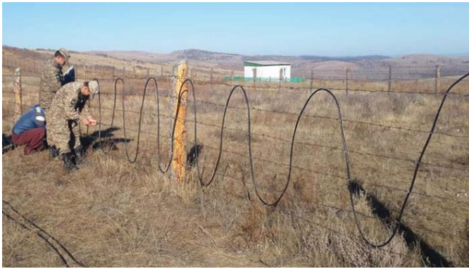
Fig. 5. Installation of Sensor Cable in the Testbed Experiment in Real Field
