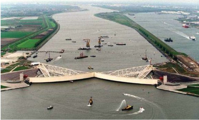
Fig. 2: The Maeslantkering Closed [9]
