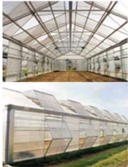
Fig. 1. Panel articulated greenhouse
